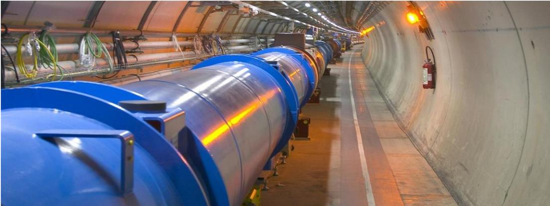
*The LHC is the most powerful accelerator ever built. The accelerator sits in a tunnel 100 meters underground. The LHC pushes protons or ions to near the speed of light. It consists of a 17-mile ring of superconducting magnets with a number of accelerating structures that boost the energy of the particles along the way.*
